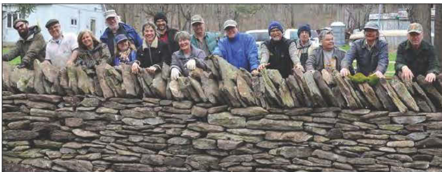
Neighbours working together on the Morrison Point Dry Stone Wall Project.
